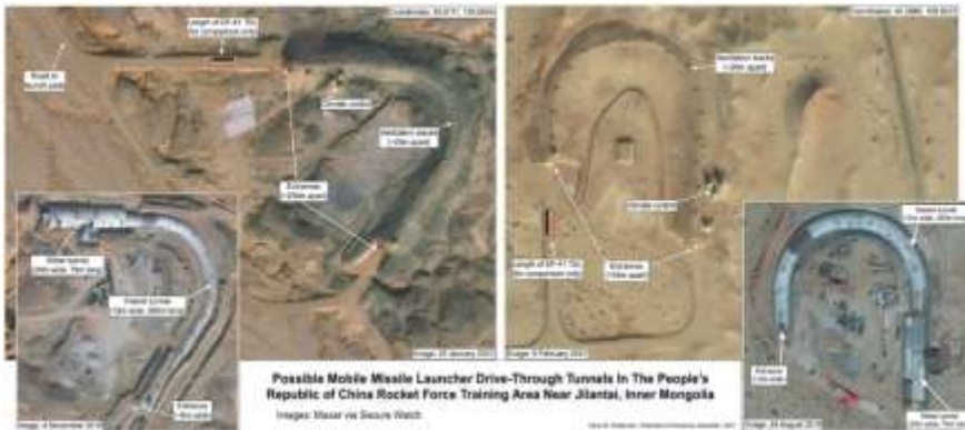
Figure 7. Works on the construction of a facility for portable rocket launchers
